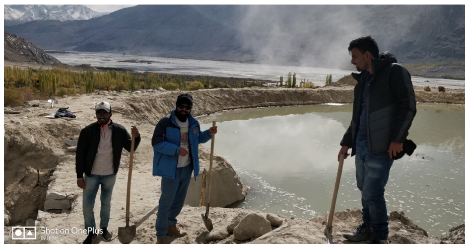
The interns working on a site
