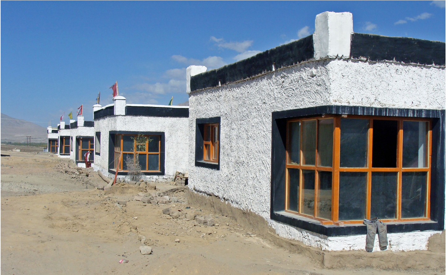
Passive Solar Rehabilitation project at Palam
